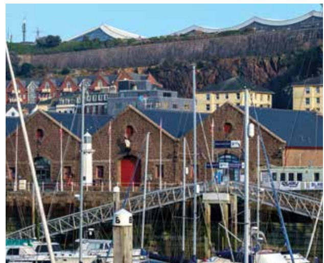
Replacement Maritime Museum roof.
