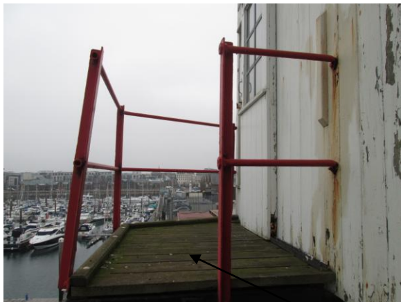
Surface build up causing slipping hazard
