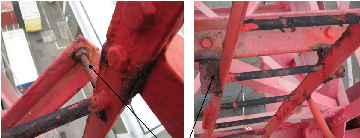
Corroded ladder section fixings and fasteners
