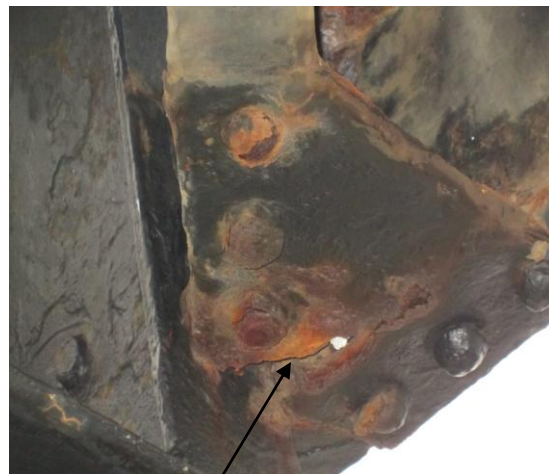
Fracture to one joining plate
