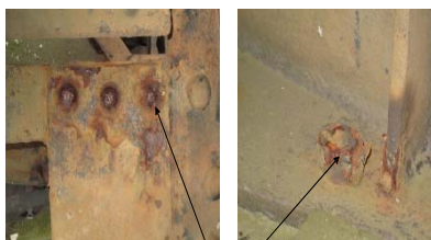
Bolts and fixings are completely rusted through making them ineffective.
