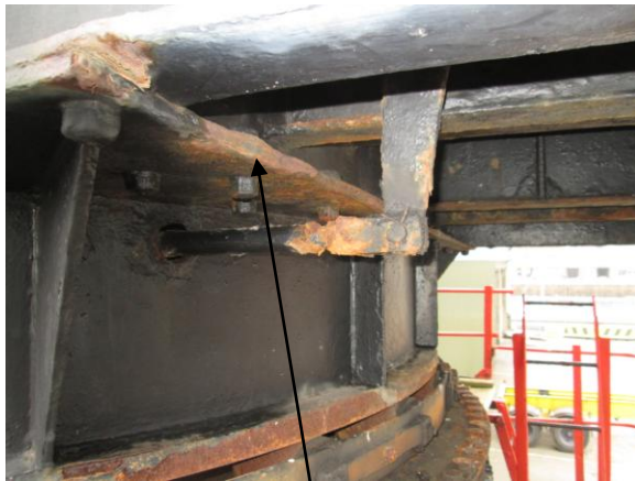
Corrosion to load bearing components
