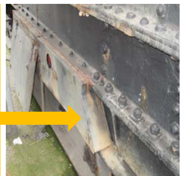
There are significant signs of collision damage to several major elements, other components are warped and twisted, causing considerable Health & Safety issues .
