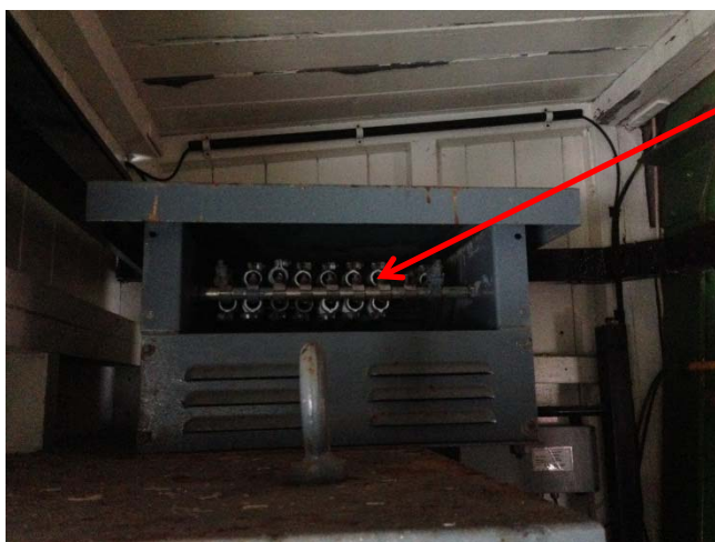
Figure 9 - Resistors with asbestos rope heat lagging
